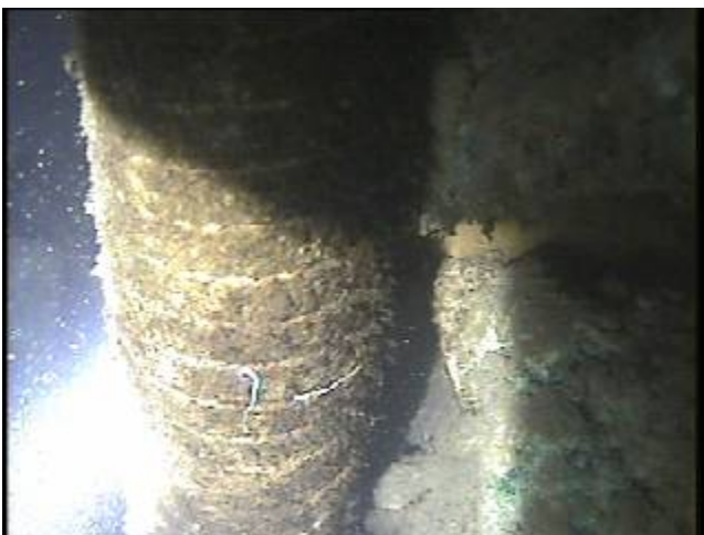
Figure 38. A lagged pipe on the starboard side of the conning tower, shows lagging – presumably asbestos - in excellent state of preservation.
